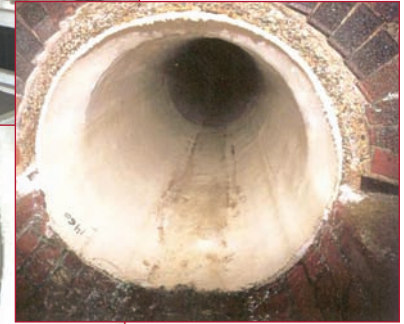
The rehabilitated pipe.
