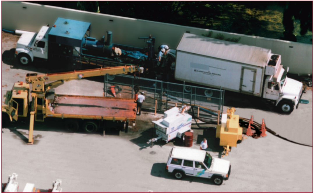
The critical pipe line rehabilitation at Westwood Lakes
